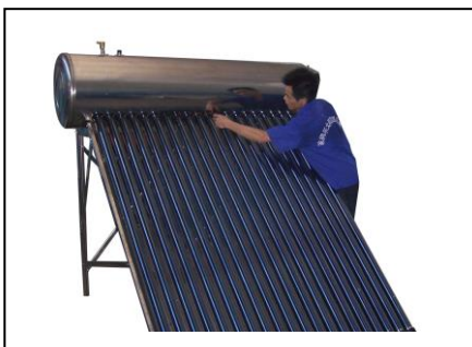
Check Anti-dust Rings to make sure they seal tank well
